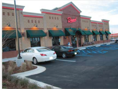
The new Demos' restaurant in Florence, Alabama, for which Dan designed much of the exterior.
